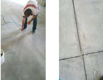
CLEAN THE SURFACE AND THE JOINT
